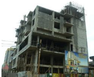
CBO Building in Nekemte (Currently under Construction)
