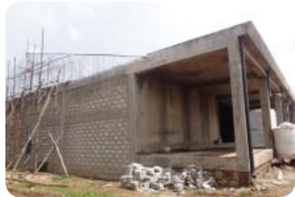
Plant under construction
