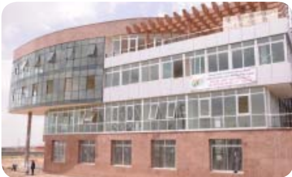
OCFCU office complex
